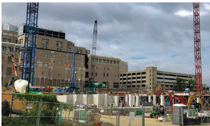
Cincinnati Critical Care Building construction site, Erkenbrecher and Burnet Ave.
